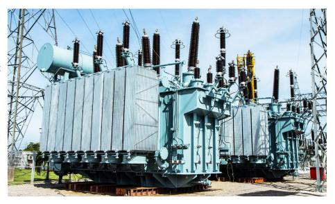
**Solution:** Using ShockLog 298 recorders, the company recorded direction, amplitude, and duration of impact forces to their transformers to determine that low frequency impacts (duration > 50 milliseconds) during transport were causing failure. Capturing the acceleration (waveform) and impact duration helped the company to both make product design improvements and set alarm threshold levels to monitor the product while in transport and avoid the costly installation of damaged product.
